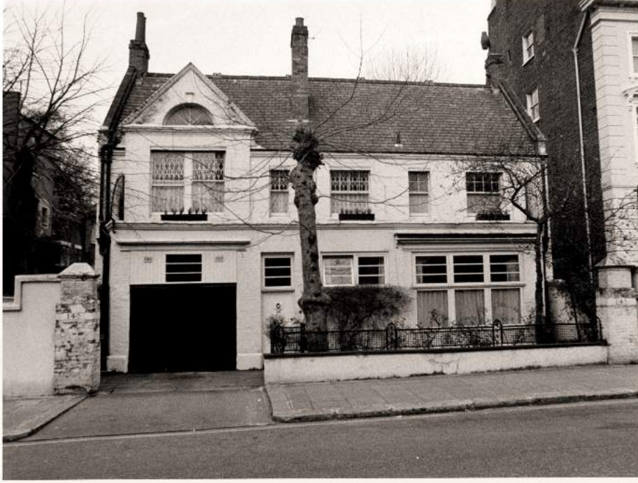
Pembroke Crescent 14A
