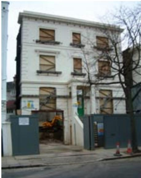
A case in point is No 14 Pembridge Place where it would appear that the whole of the building behind the front facade has been demolished.
